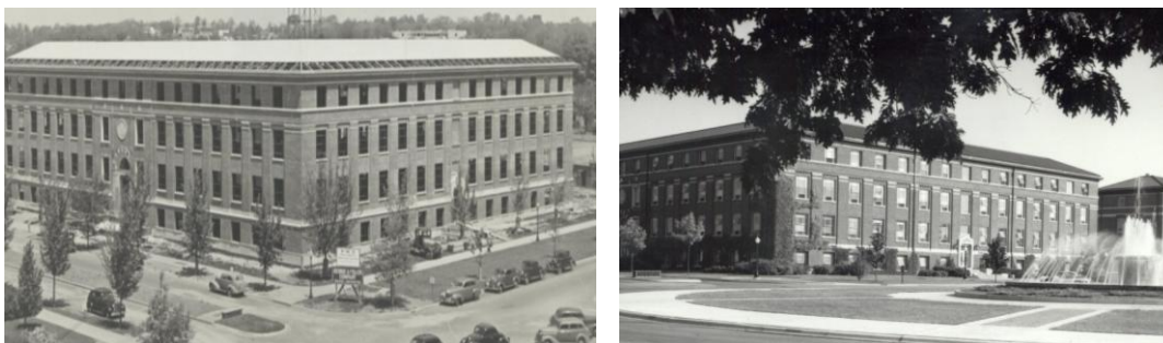
The CMET building in May 1940 ( left ) and in 1985 ( right ).
