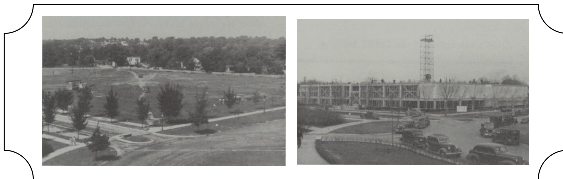
The site of construction of the CMET building in 1938 ( left ) and 1939 ( right ).
